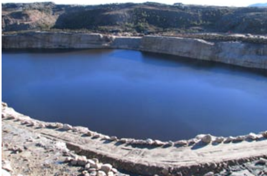
The $14 million Mangatini Sump at Stockton holds up to a million cubic metres of water and sediment. Photo: Solid Energy.
