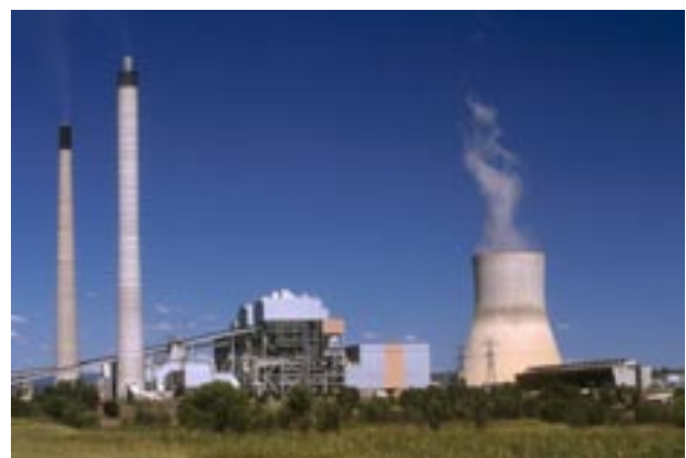
The Callide A station is home to the Oxyfuel Project. The old station was refurbished in 1998 and mothballed in 2000 for this project - one of the units was recommissioned in 2009. Photo: David Brown, CS Energy.
